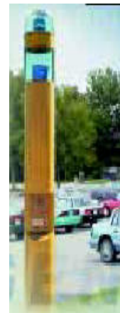
Figure 14: Emergency Call Box
