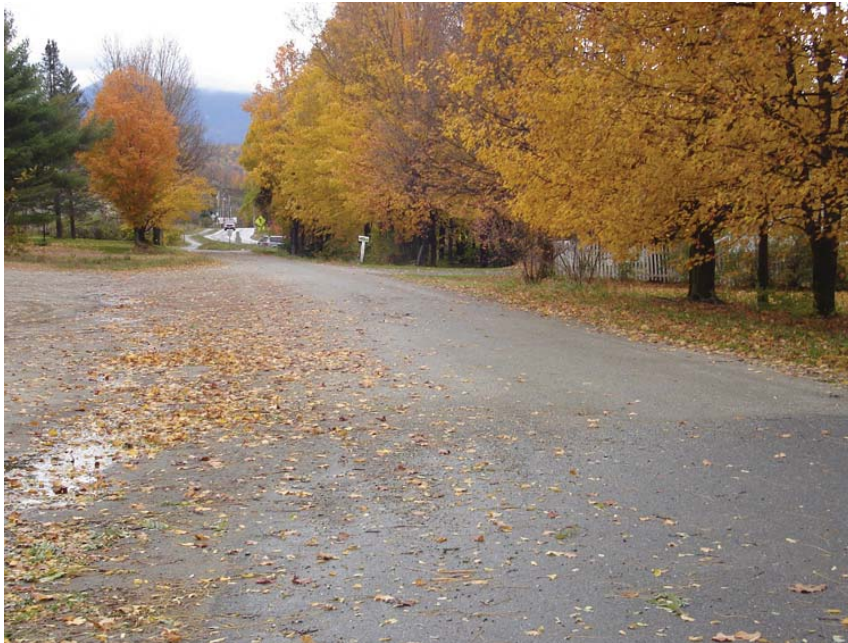
Figure 2: Dickinson Street (Looking East)
